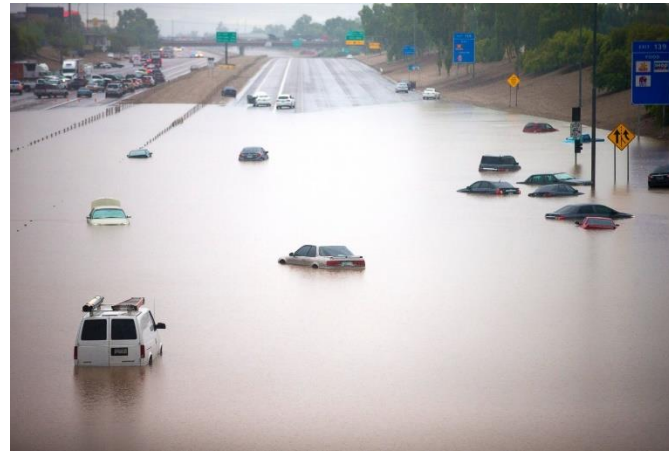
I-10 Flood in Phoenix, 2014
